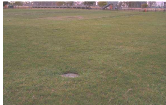
The picture above is an example of a sprinkler cover. This picture does not reflect the actual cover or conditions referred to in this case study.
